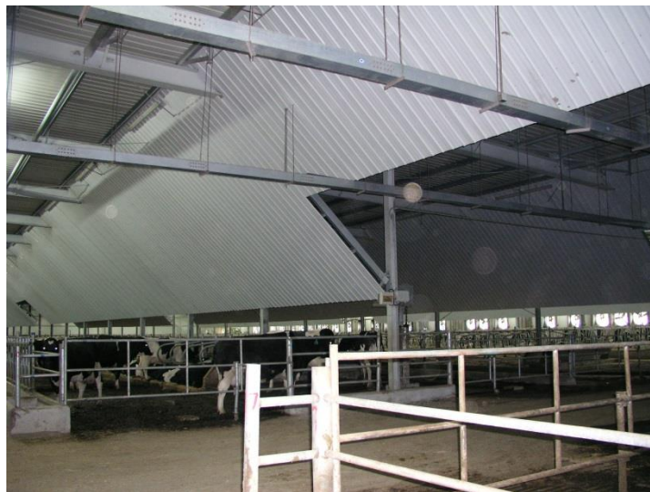
FIG. 6. Slanted baffle in cross-ventilated barn. Higher air velocity is often observed in cross alleys where baffles are higher to allow equipment to pass underneath.
